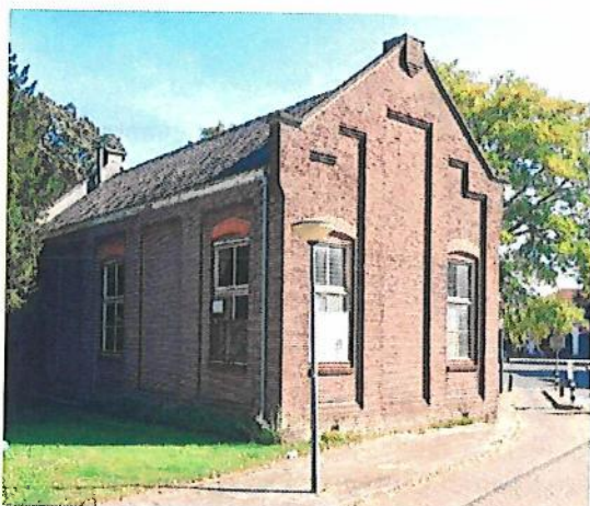
Te slopen gymzaal
